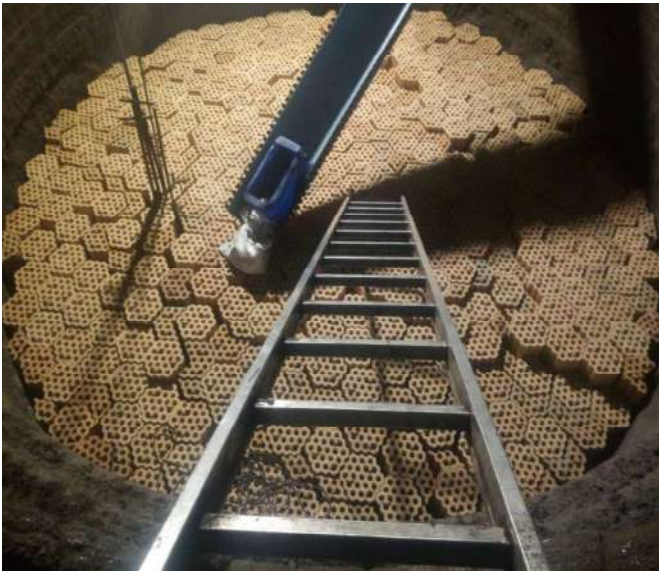
Figure 3. The stove after refractory knitting.
