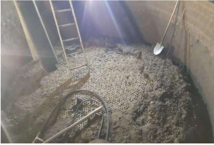
Figure 2. Brick appearance of the stoves after slag cleaning
