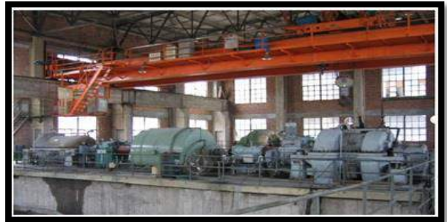
Figure 6. The TRT that is installed for a BF with a volume of 380 m 3 (Anonymous, 2009)
