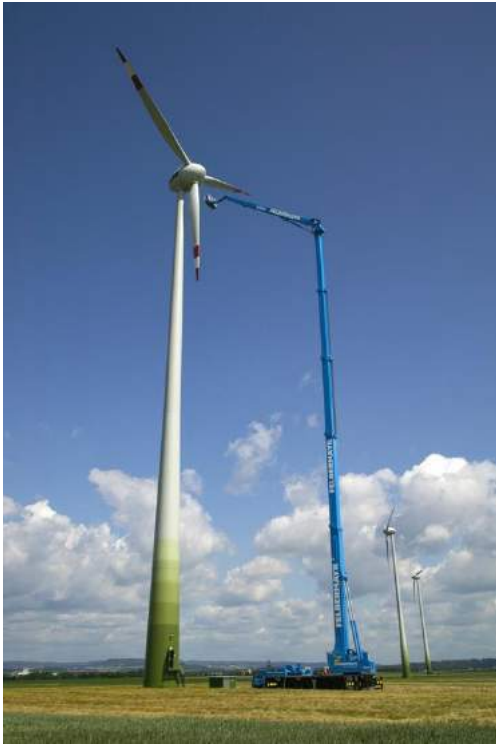
Fig.2 Maintenance of wind turbine with an aerial work platform
