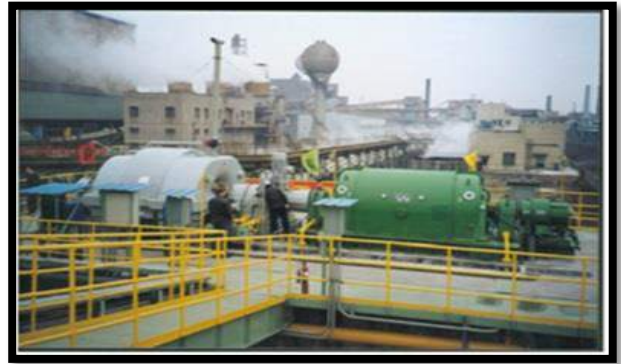
Figure 5. The TRT that is installed for a BF with a volume of 2500 m 3 (Anonymous, 2003)
