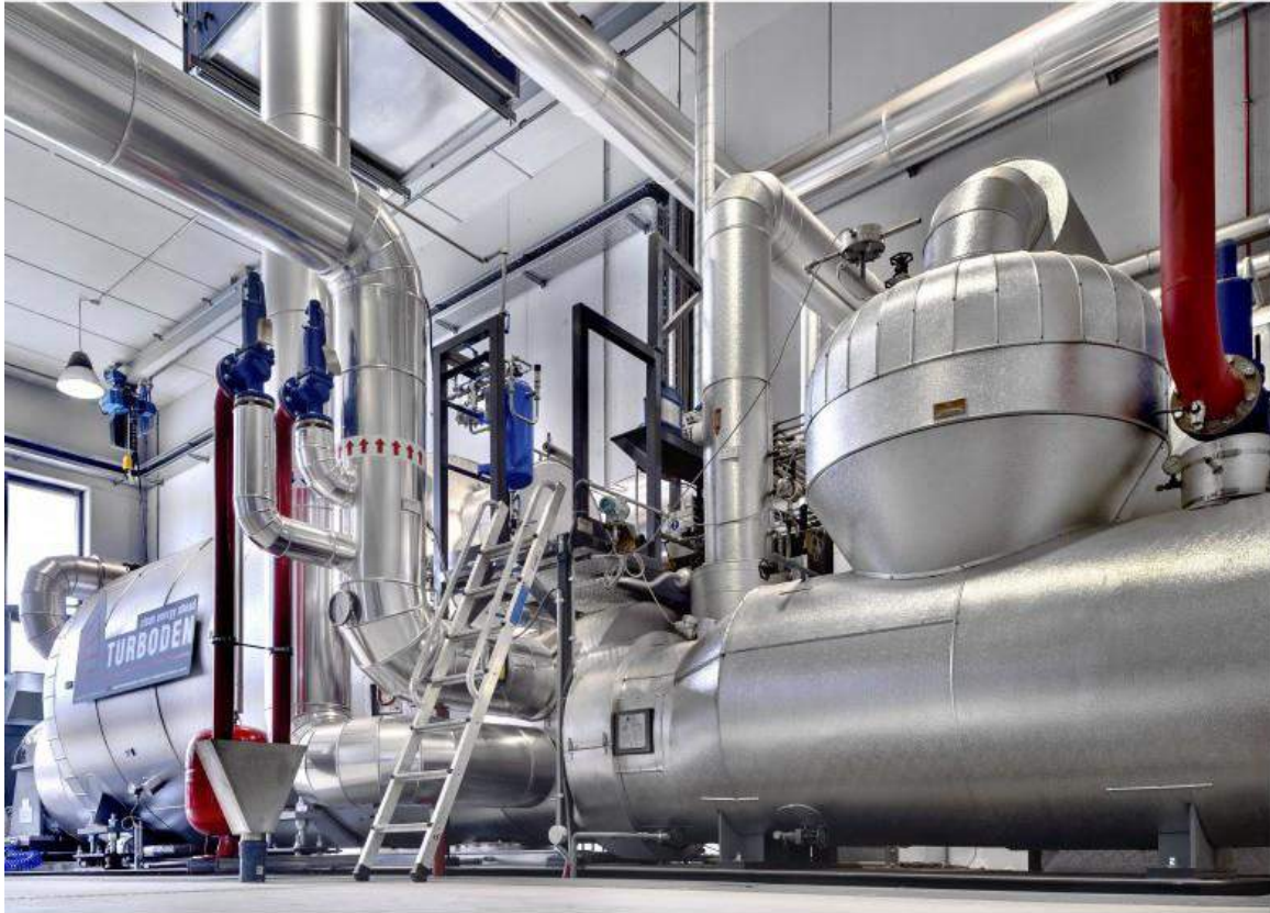
800 kW biomass ORC Turboden plant for Teleriscaldamento Varna-Bressanone. Varna – Bolzano, Italy - 2008
