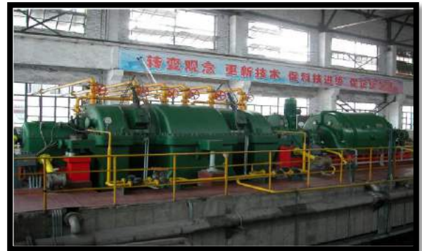
Figure 7. Generator Application for two BF with a volume of 2x450 m 3 (Anonymous, 2010)
